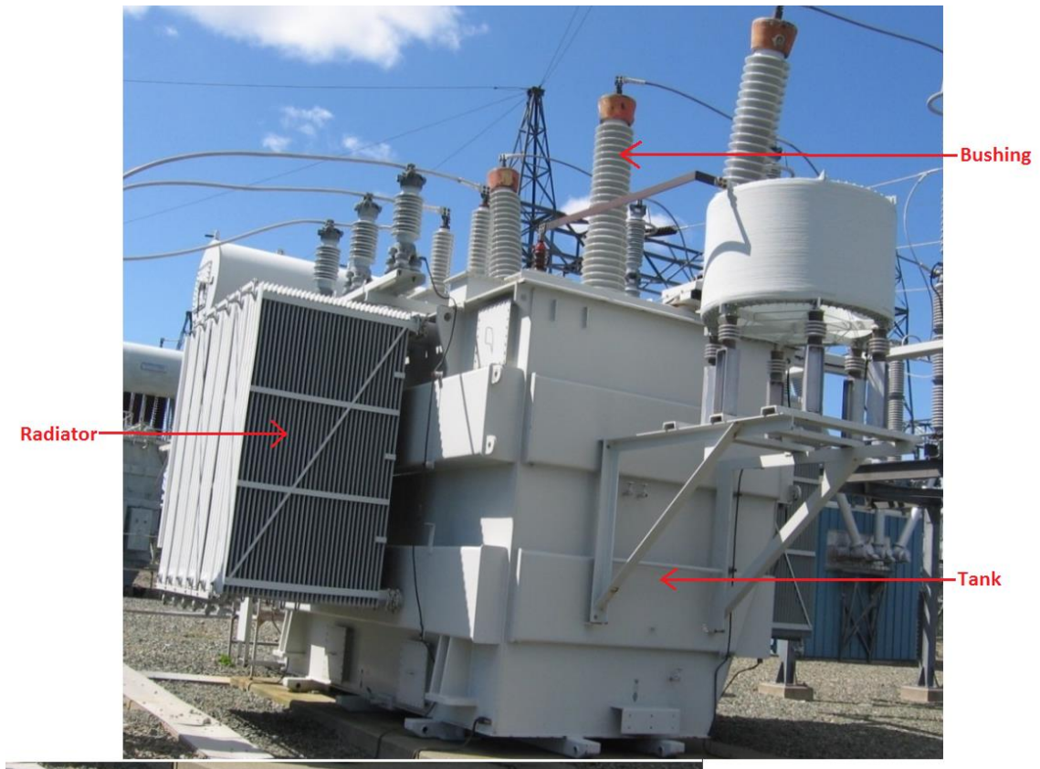
Figure 8: Power Transformer
